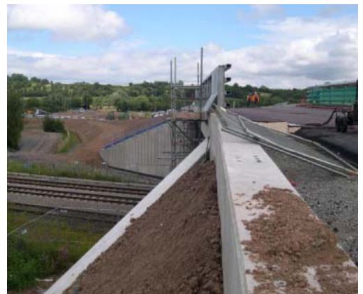
New Leominster railway bridge nearing completion.
